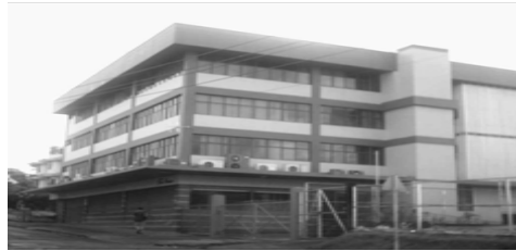
▶ Headquarters for Ministry of Health
